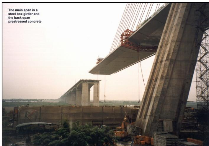
An economic design of a cable-stayed bridge requires that the bending stiffness of the bridge deck is used to achieve an efficient distribution of the loading to the stay cables. On this bridge it was achieved by imposing an appropriate pre-deformed shape to the whole bridge deck.
