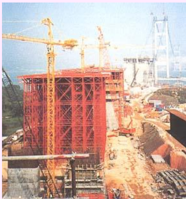
Massive falsework system was among the largest ever erected
