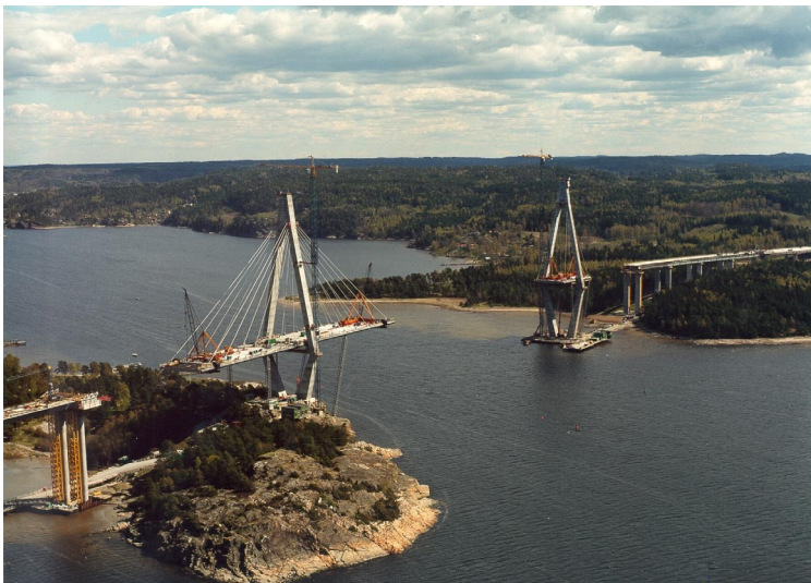
Fig. 5 Typical construction stage for stayed cable bridge
