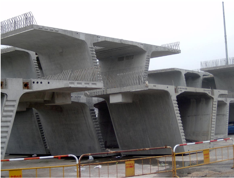
Fig. 4 Segments waiting for erection
