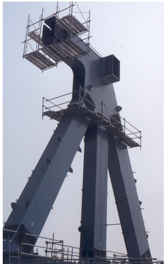
Fig.5 Portal frame under construction
