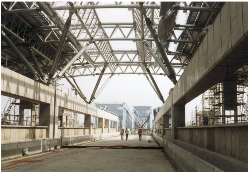
Fig.1 T'aichung station and adjacent steel truss bridges.
