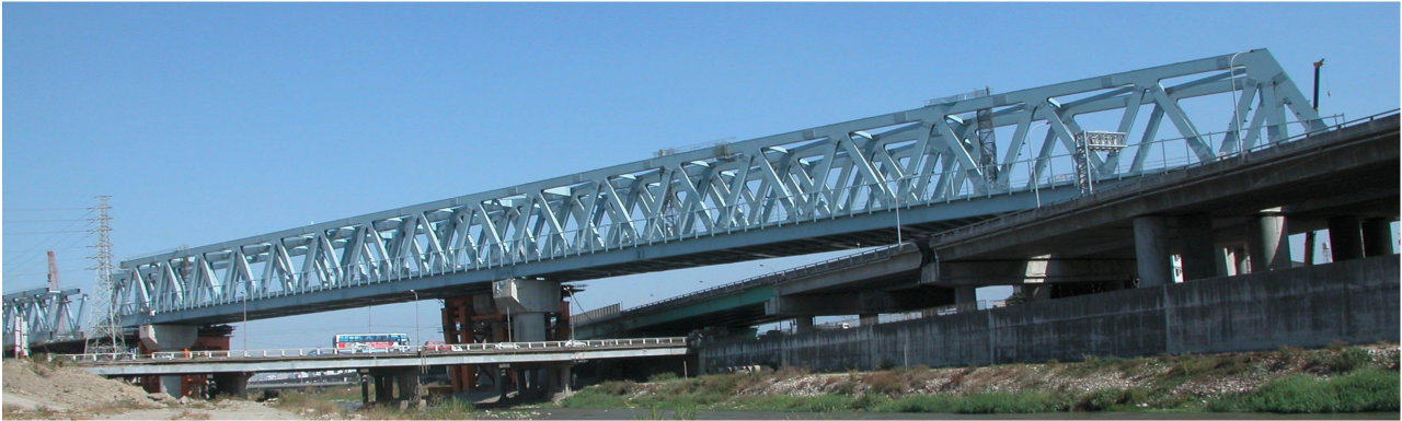
Fig. 3 Three span steel truss under construction
