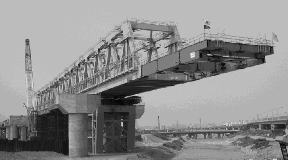
Fig. 1: Launching of a 3-span truss bridge.
