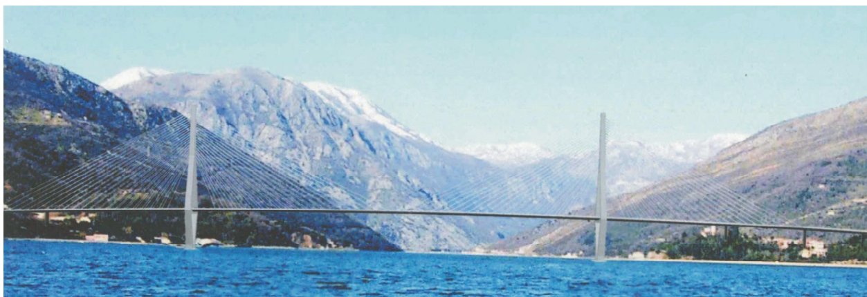
Fig.13 Verige Bridge, spans of 41+50+90+130+450+130+90m, Montenegro [4]
